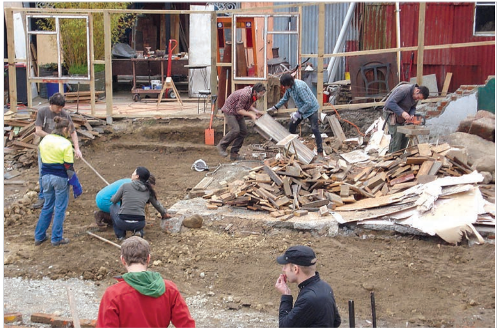
PHOTO 8. Community members participating at a working bee building the Petanque Court.
