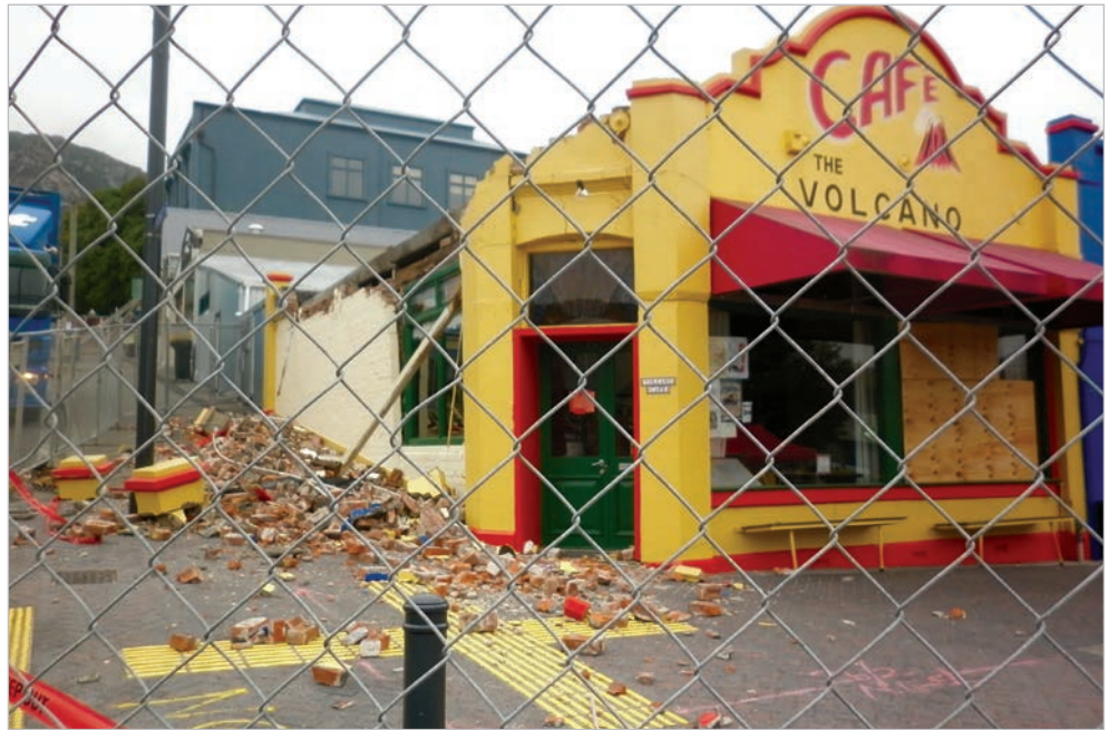
PHOTO 5. Significant damage to local businesses was caused by the earthquake.
