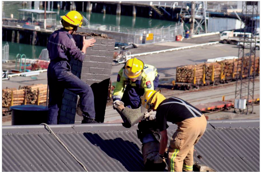
PHOTO 4. Lyttelton Fire Brigade dismantling a dangerous chimney.
